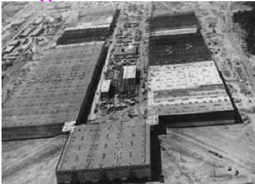
ORNL K-25 Gas diffusion plant (1/2 mi long) Manhattan Project
