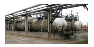
Two steps de-salter operates in DR CDU units Average calt content of crude: 20-40 ppm Aim: <4 ppm Less water request
